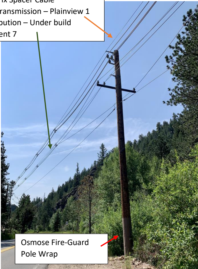
Three-Phase Covered Conductor Blue Mountain 2
