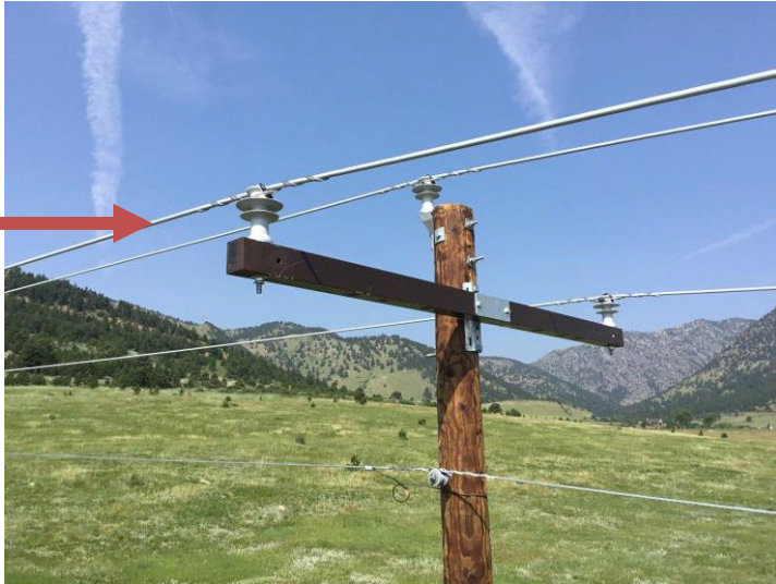
Three-phase covered conductor. (Blue Mountain 2)
