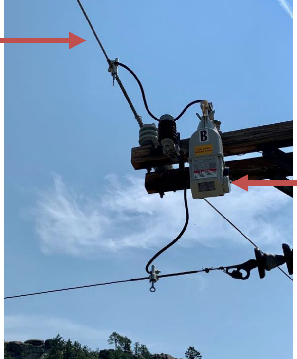
New covered conductor. New 'smart' recloser for isolating power lines.
